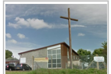
Yeovil Methodist Church at Chelston Ave
