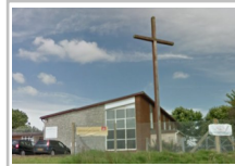
Yeovil Methodist Church at Chelston Avenue
