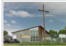
Yeovil Methodist Church at Chelston Avenue
